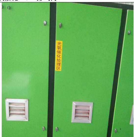
喷漆工序过滤棉+光氧催化+15m 排气筒
